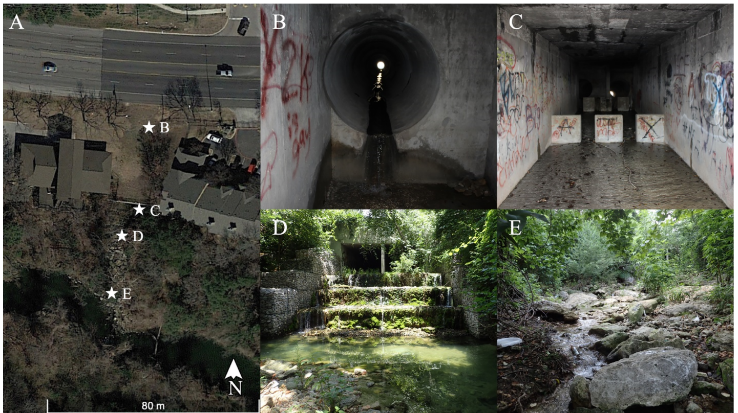
Figure 2 Descriptive site images of Brushy Creek Spring. (A) Aerial image (Google Earth imagery) of Brushy Creek Spring in Round Rock, Williamson County, Texas. Stars designate the locations of photographs B–E. All photographs face upstream. (B) Junction of culvert tunnel under US79 and box culvert with groundwater discharging from the PVC pipe, seams in the culvert tunnel junctions, and at seams and cracks at the culvert tunnel and box culvert interface. (C) Right side of the box culvert upstream of the gabion with shallow, spring water sheet flowing across concrete bottom. (D) Downstream entrance of box culvert, gabion, and pond. (E) Spring run downstream of gabion (Photographed by Zach Adcock).
