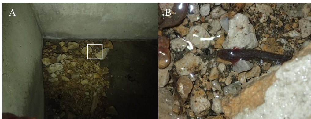
Figure 5 Jollyville Plateau Salamander ( Eurycea tonkawae ) capture location at Brushy Creek Spring. (A) Groundwater discharges from cracks in the concrete along the culvert wall and floor junction and from the nearby spring diversion PVC pipe. White square outlines the area in photo (B). One E. tonkawae partially covered by a large cobble (Photographed by Zach Adcock).
