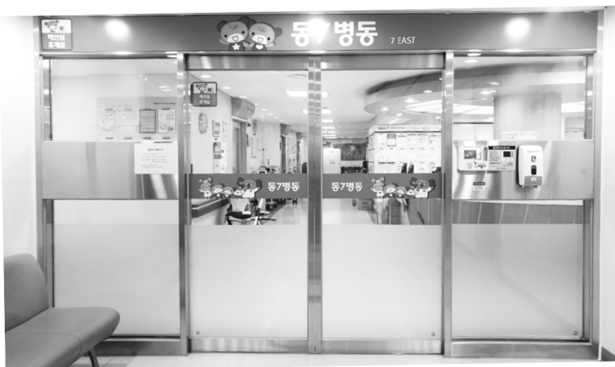
Fig. 1. Glass sliding door of a pediatric ward (before intervention).
