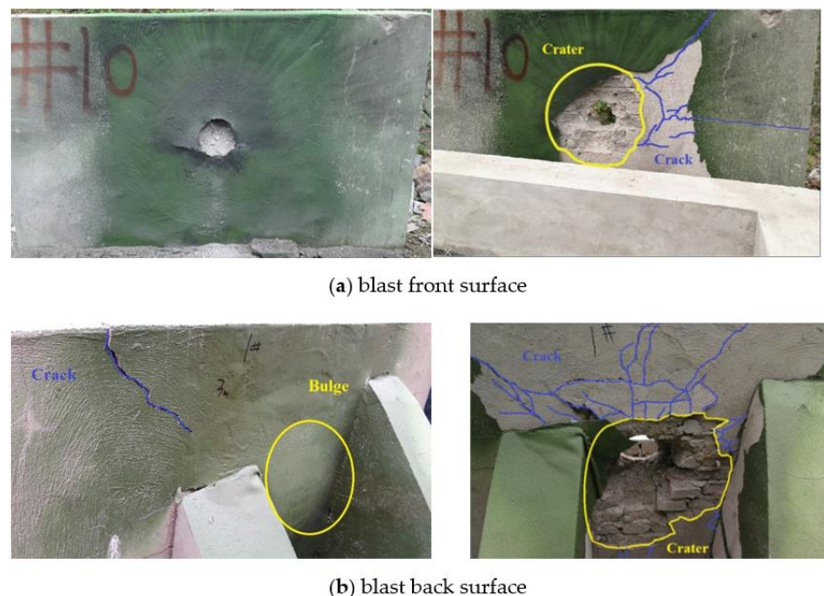
Figure 7. Damage to the reinforced 240 mm wall in the test.
