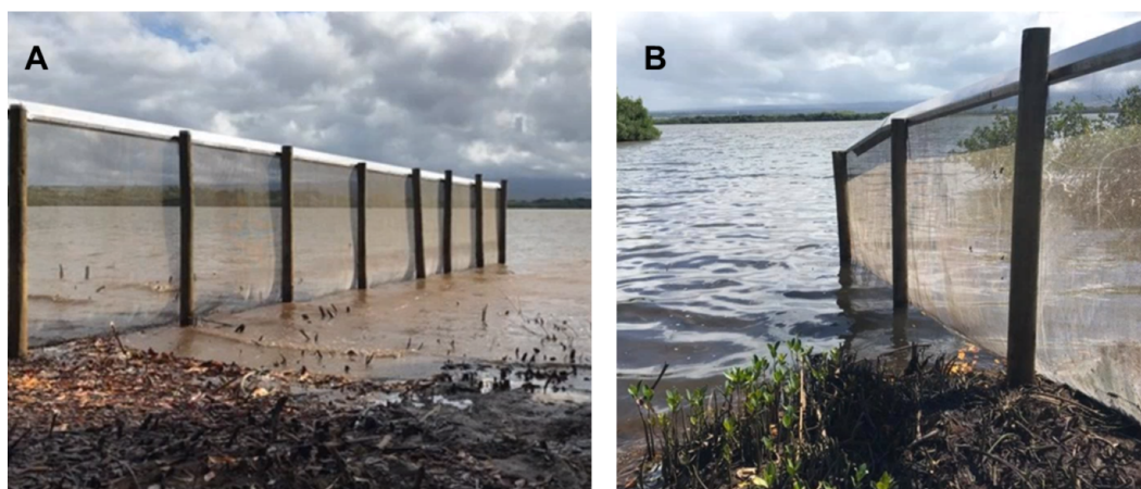
Figure 4 The west (A) and east (B) ends of the exclusion fence extending into Pearl Harbor, using the water as a natural barrier to exclude mammalian predators. Photos were taken within an hour of each other on the same day by Lindsay Young at medium tide.
