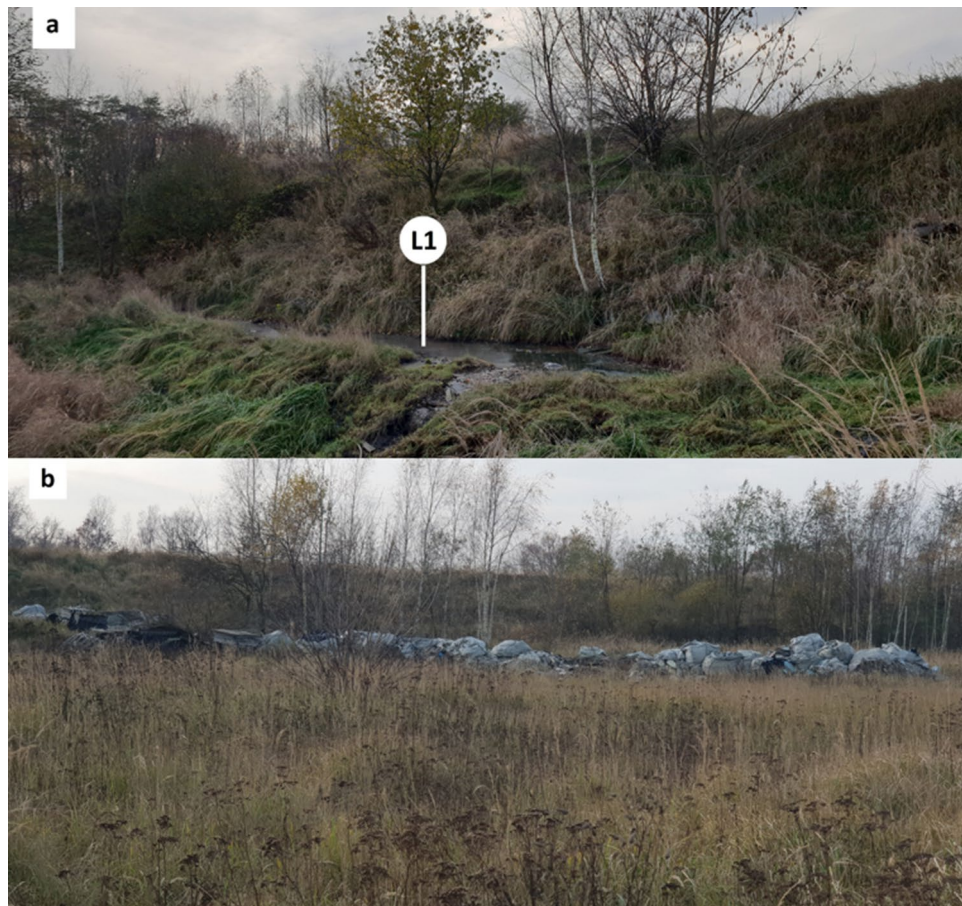
Figure 2. The closed landfill for hazardous waste of the former "Boruta" Dye Industry Plant with visible plant succession. The slope of the landfill near the leachate accumulation site L1 (a) and the surface of the landfill with asbestos bags (b).
